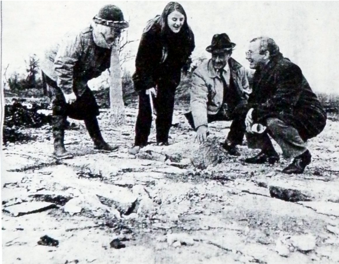
When the project began ... Pamela Whitby (WI), Gina Rowe (British Trust for Conservation Volunteers), Mr Whitney and David Williams (Shell UK) inspect the work of clearing the concrete
